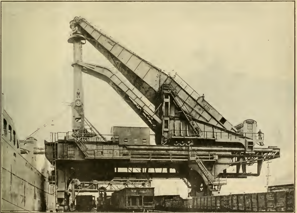
Unloader and Electric Pusher Locomotive at Claremont Terminal of Lehigh Valley Railroad
